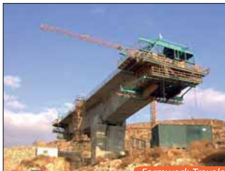
Formwork Traveler
