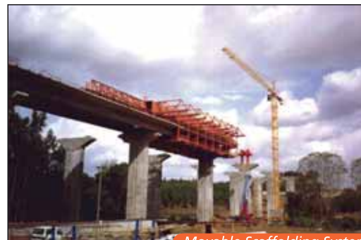
Movable Scaffolding System
