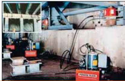
Bridge Bearing Repair & Maintenance
