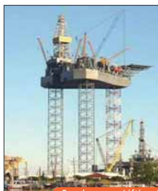
Synchronous Lifting & Weighing System of Oil Rig
