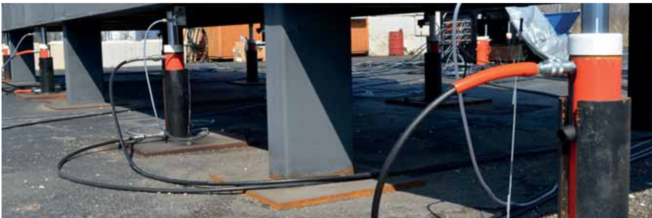
Below: Positioning of HVAC equipment during installation.
