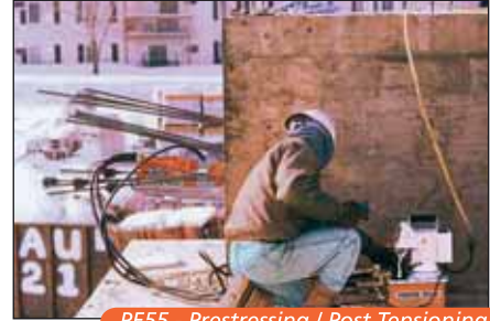
PE55 - Prestressing / Post Tensioning
